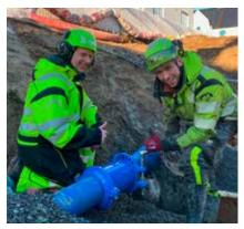
"The Supa One<sup>™</sup> coupling is very easy to install. Tightening with a standard power tool and torque wrench to 150 Nm works very well." - Kaare Mortensen A/S, Norwegian construction company.
