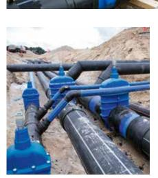
**Flexible material**PE pipes are flexible and follow the terrain, so there is no need to level the soil in the trench.
